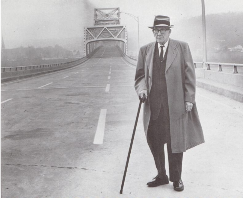
Congressman Brent Spence on the Brent Spence Bridge Prior to Opening, 1963. Photo Credit: Jack Klempe
